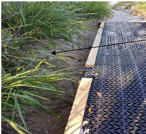
Entry point when storm water from pit at road head overflows across dune into access way. Previously reported to Council with pics “erosion from storm water as a safety risk.
