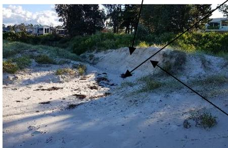
Storm water discharged from Storm water pipes through the dune cause erosion.
